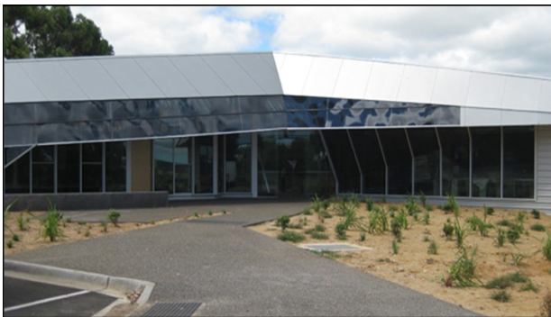
The New Campus was built on a Greenfield site in Nerrena Road, Leongatha (South Gippsland)
